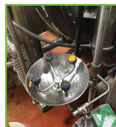
CAN'T RUN SHOWER & EYEWASH SIMULTANEOUSLY
